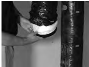
Insert insulation inside the double collar.
