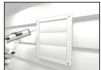
**1** Using the duct connection of the outside hood, outline the intake & exhaust holes to be cut. The holes should be slightly larger than the duct connection to allow for the thickness of the insulated flexible duct. Cut a hole for both the intake and exhaust hoods.
