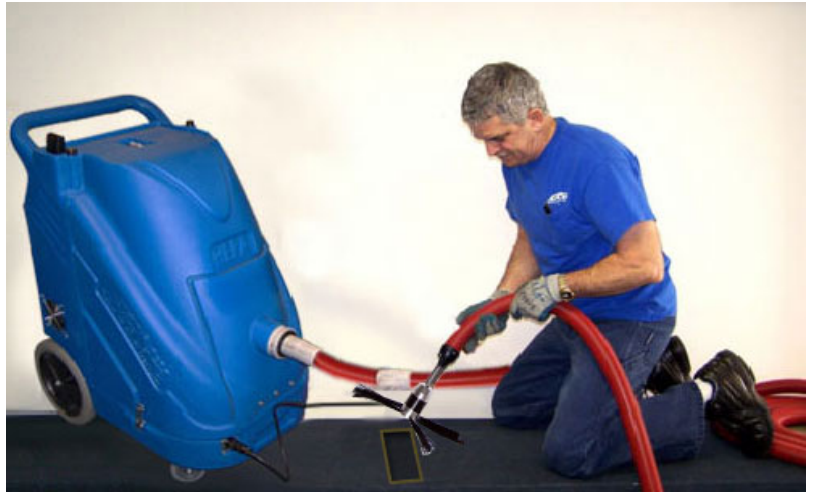
Cleaning Floor Ducts
