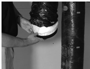
Insert insulation inside the double collar.
