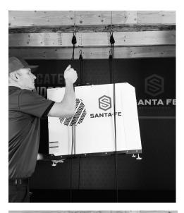
**Step 5:** Once the dehumidifier is at the height desired, use a level to make sure it is even on both sides and front to back.
